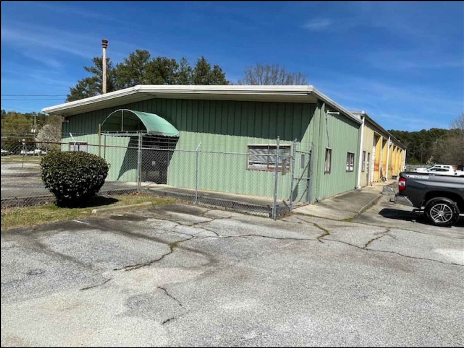
Large Pre-Engineered Metal Building (7,250 SF)
