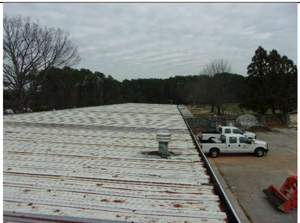
Black roof sealant around vent
