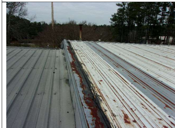
Asbestos containing Black roof sealant along roof seam
