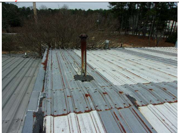
Black roof sealant around vent
