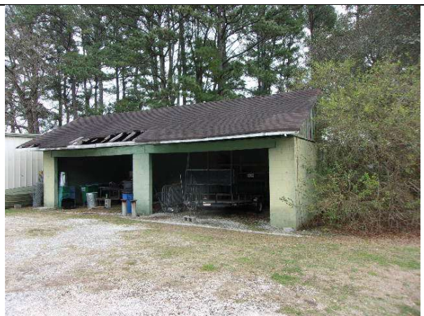
Open equipment storage building—failing roof
