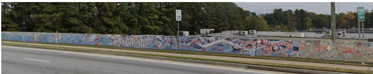
Mural Painted on Highway 78 Eastbound Concrete Retaining Wall
