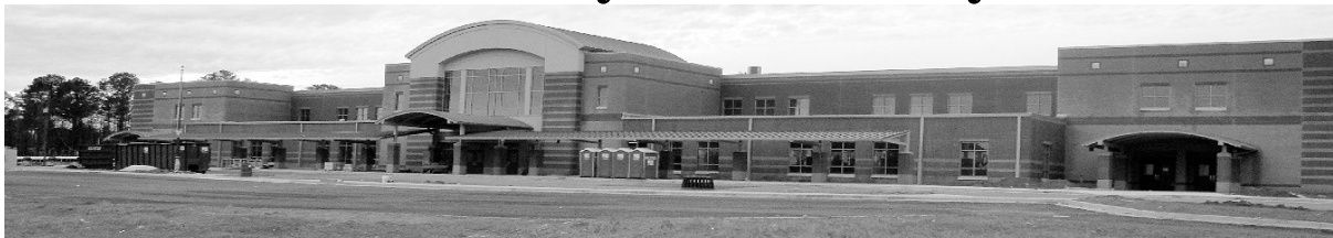
The new Anderson-Livsey school under construction
